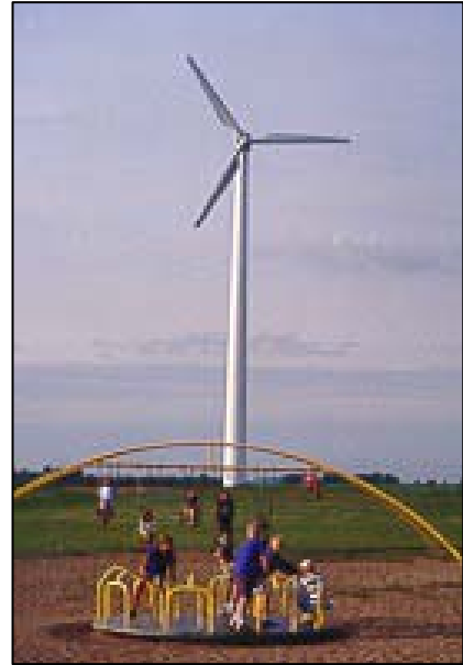
Community-owned wind turbine in Spirit Lake, IA
