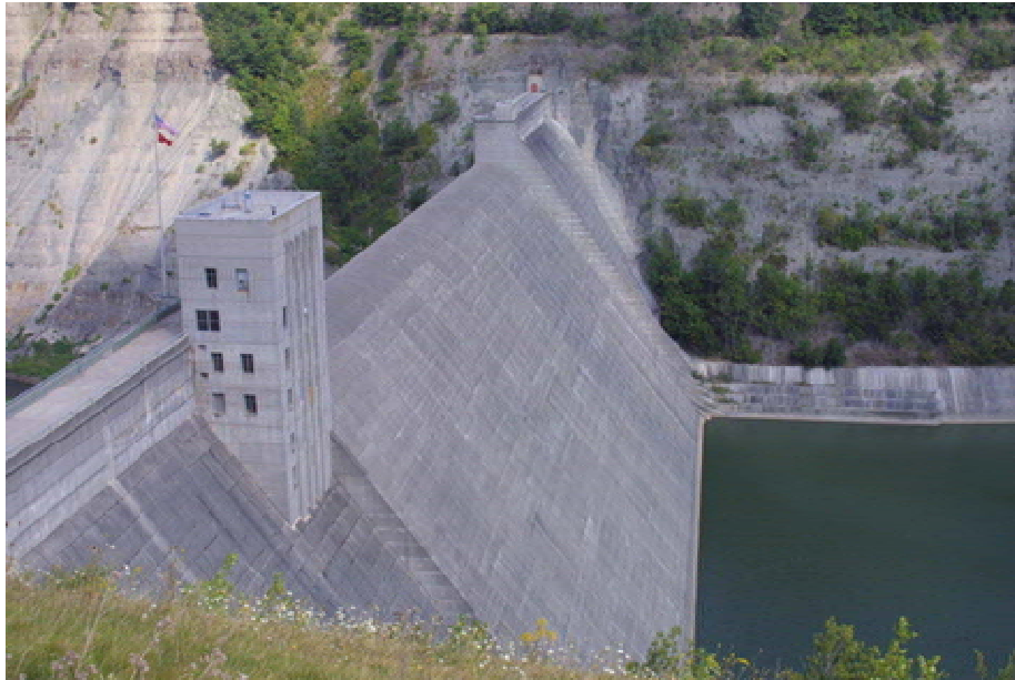
A dam on the Genesee River in New York State.
